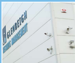
Network & External CCTV
